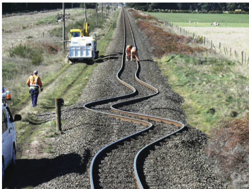
Figure 4. Train tracks in Canterbury, New Zealand, that buckled after an earthquake in 2010, in a shape that resembles the graph of w_2(x) .
